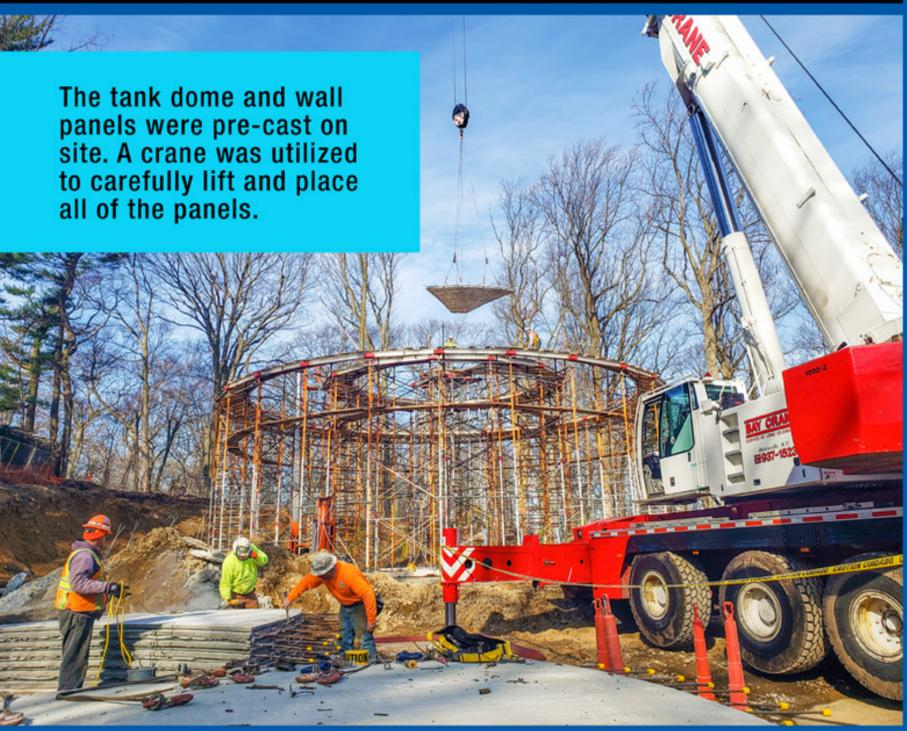
The tank dome and wall panels were pre-cast on site. A crane was utilized to carefully lift and place all of the panels.
