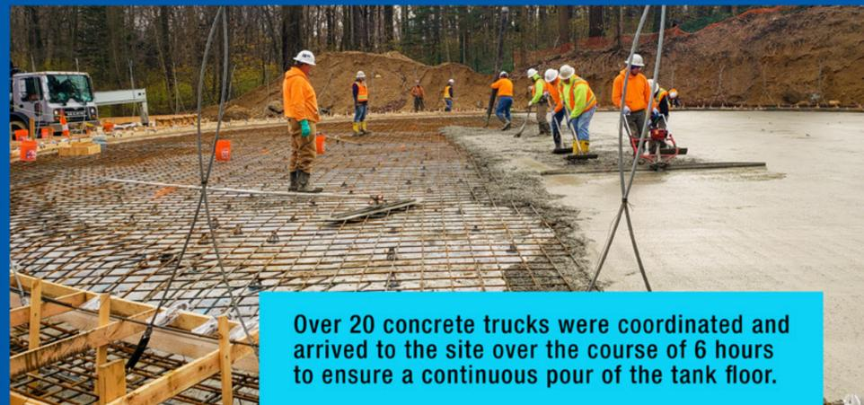
Over 20 concrete trucks were coordinated and arrived to the site over the course of 6 hours to ensure a continuous pour of the tank floor.
