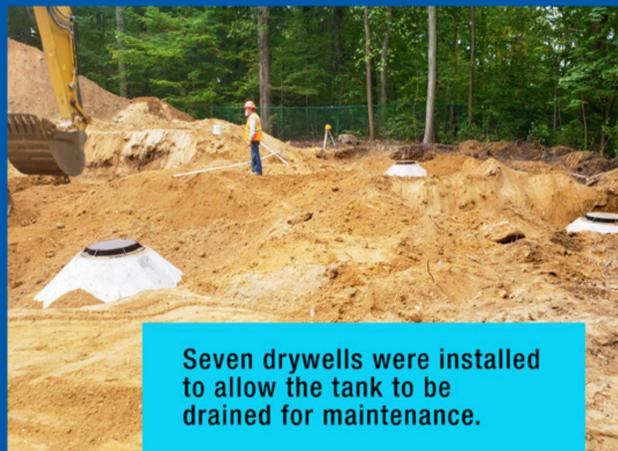
Seven drywells were installed to allow the tank to be drained for maintenance.
