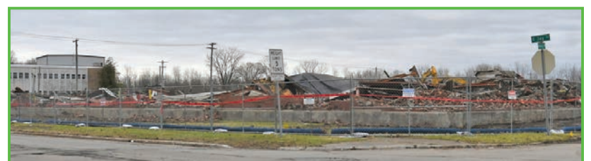
Project Blue Crab, Redevelopment Construction Activities (circa 2020)
